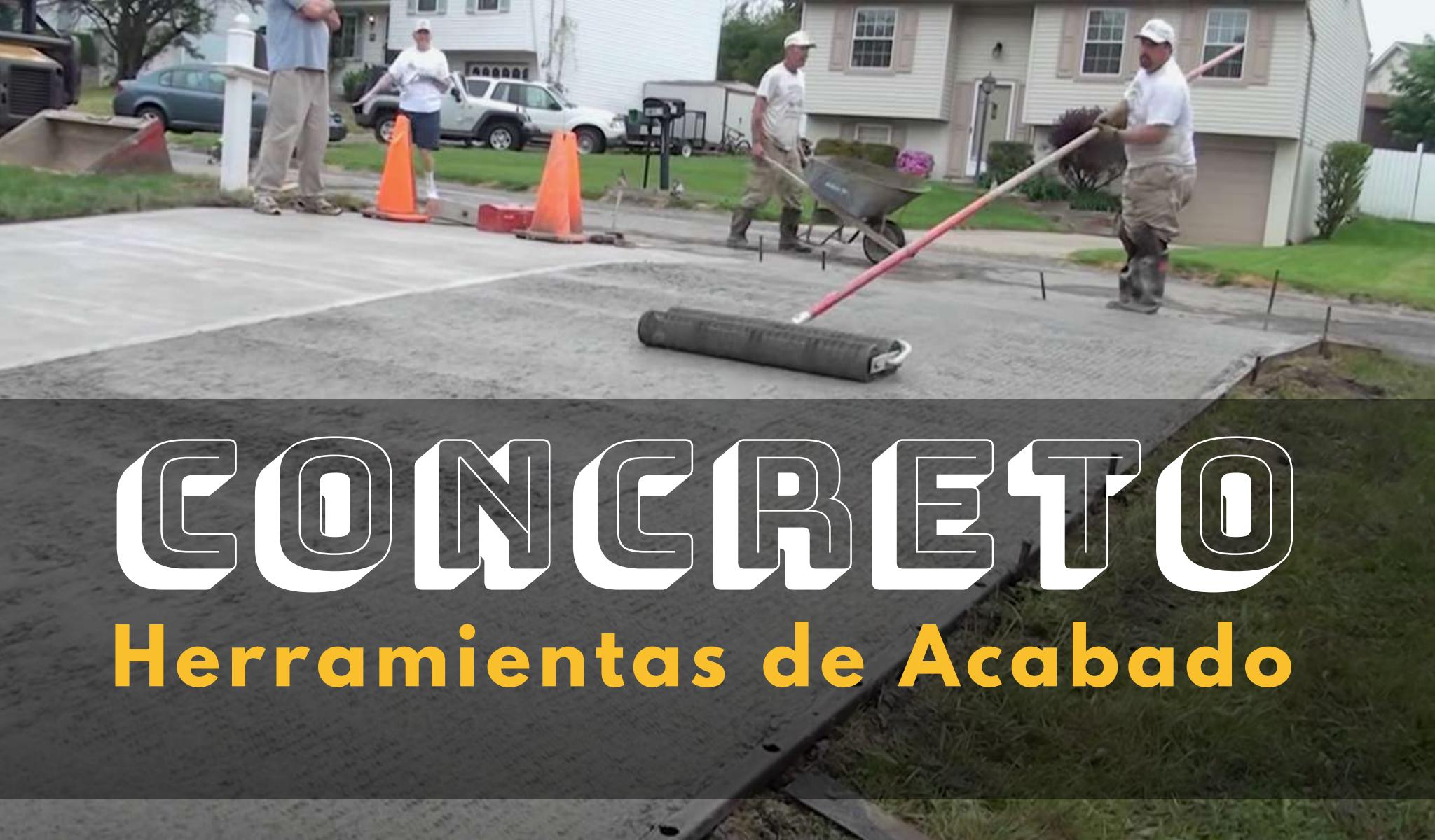
A photograph showing four construction workers on a residential street. One worker in the foreground uses a long-handled edger to smooth the edge of a new concrete driveway. Another worker with a wheelbarrow stands behind him. Two other workers stand further back, one holding a clipboard. Orange traffic cones are placed along the edge of the driveway. A house and a car are visible in the background.
